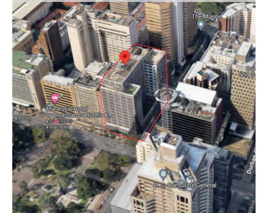
Aqua Sky Towers (Durban, SA) Commercial Offices
